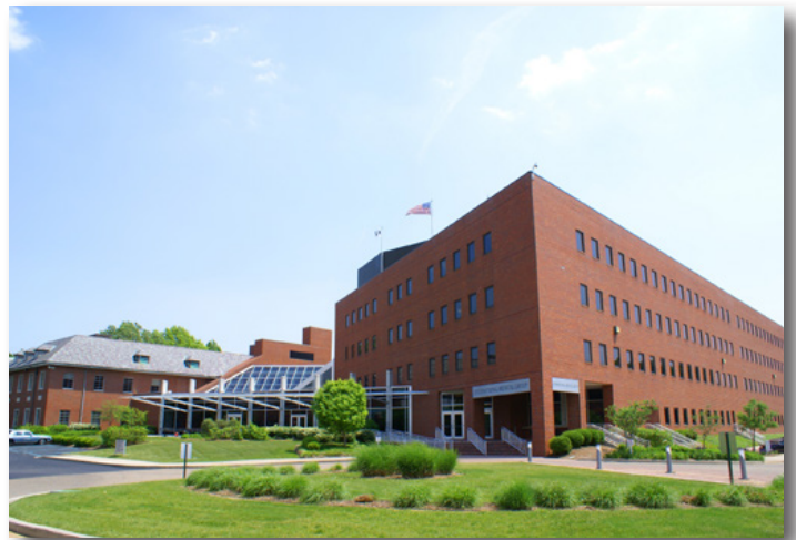
IMG World Headquarters, Indianapolis, Indiana
